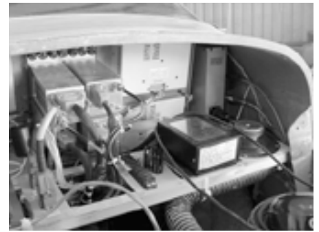
Behind the panel
