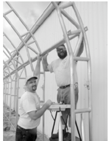
Brendan and Allen King working on Quonset building
